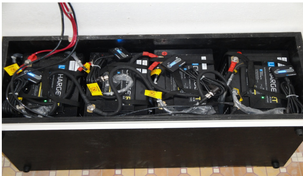
Figure 5: Valence Lithium Polymer batteries with Battery Discharge Indicators
