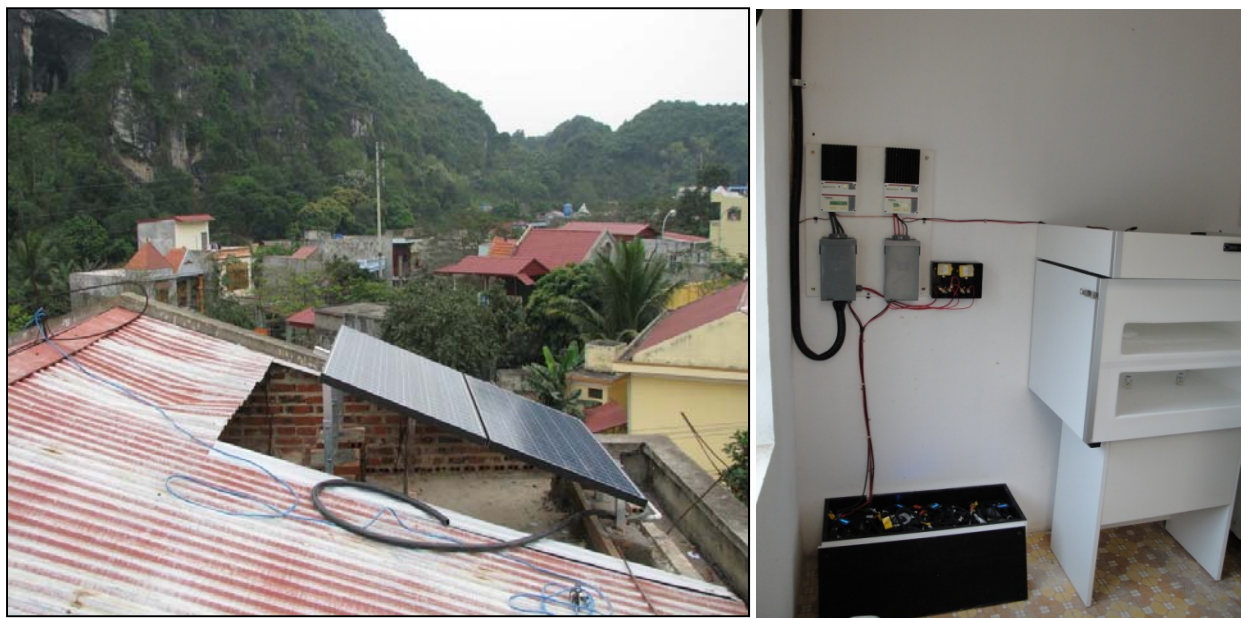
Figure 1: Cat Ba solar vaccine refrigeration installation in progress (with Valence Li Battery)
